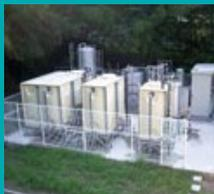
This is a groundwater membrane filtration system perfect for customers requiring a large amount of drinking water, such as hotels, hospitals and food processing plants. By creating a "mini purification plant" on the grounds and supplying water to an intake tank after it has passed through a stringent filtration process and chlorination, it is possible to lower the costs of supplying water by 20–30% per year. The system is also highly regarded in terms of its ability to respond to disasters.
