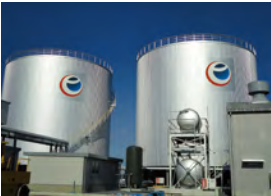
Sodegaura Asphalt Base
