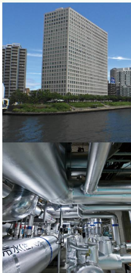
Upper right: The exterior of the building where the Hakozaiki District Heat Supply Center is located; bottom right: Underground heat supply pipes in the Hakozaiki District. These incorporate a full range of safety measures to control waterborne particulates and salt damage from brackish water.
