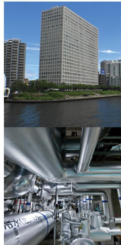
Upper right: The exterior of the building where the Hakozaki District Heat Supply Center is located; bottom right: Underground heat supply pipes in the Hakozaki District. These incorporate a full range of safety measures to control waterborne particulates and salt damage from brackish water.
