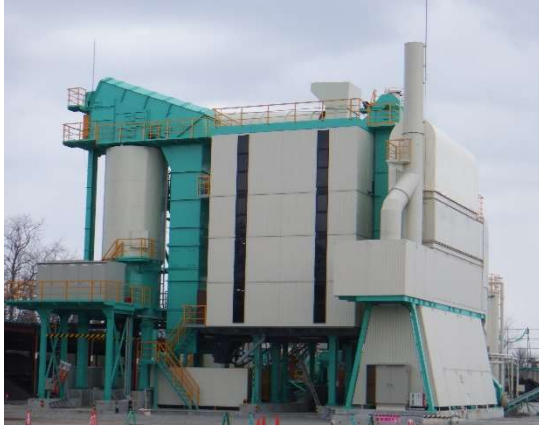
The asphalt plant
