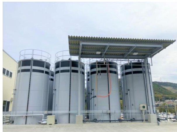
Aqueous urea storage tanks installed in Okayama Plant
