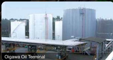
Oigawa Oil Terminal
