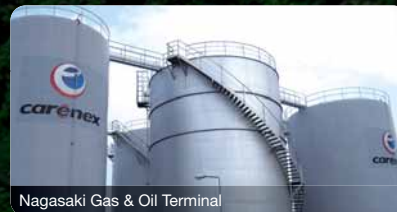
Nagasaki Gas & Oil Terminal
