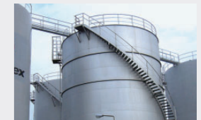
Nagasaki Gas & Oil Terminal
