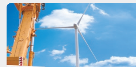
Wind power generation facility currently under construction (Tainai City, Niigata Prefecture)
