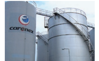
Nagasaki Gas & Oil Terminal
