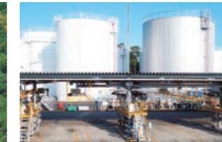
Oigawa Oil Terminal
