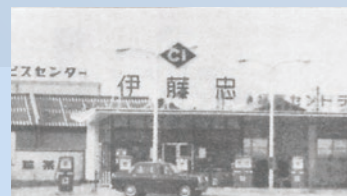
A refueling station in Fukuoka during the Itochu Fuel Corporation era
