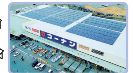
Self-consumption solar energy system installed on the roof of a Home Center Kohnan outlet
