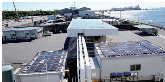
Self-consumption solar power systems installed at Sodegaura Asphalt Terminal. These are expected to realize a CO 2 emissions reduction of approx. 15% compared with conventional power.
