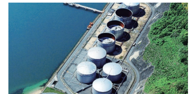
A tank terminal, the supply base for petroleum products
